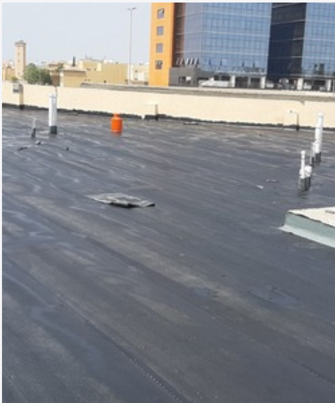
Bituminous Membrane Waterproofing - Jeddah
