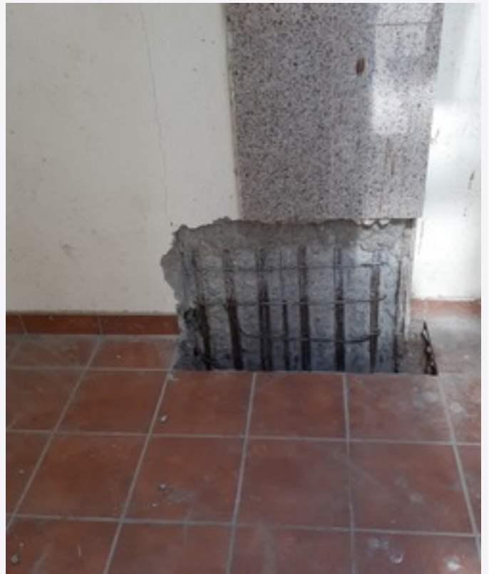
Concrete Repair Works
