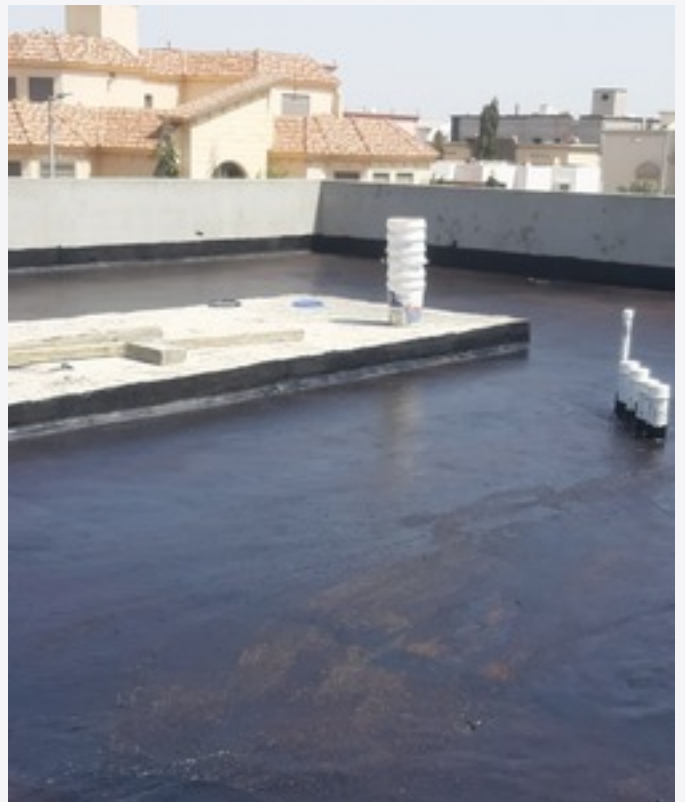
Roof Waterproofing - Prince Sultan Road, Jeddah
