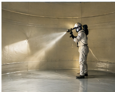
Water Tank Internal Coating
