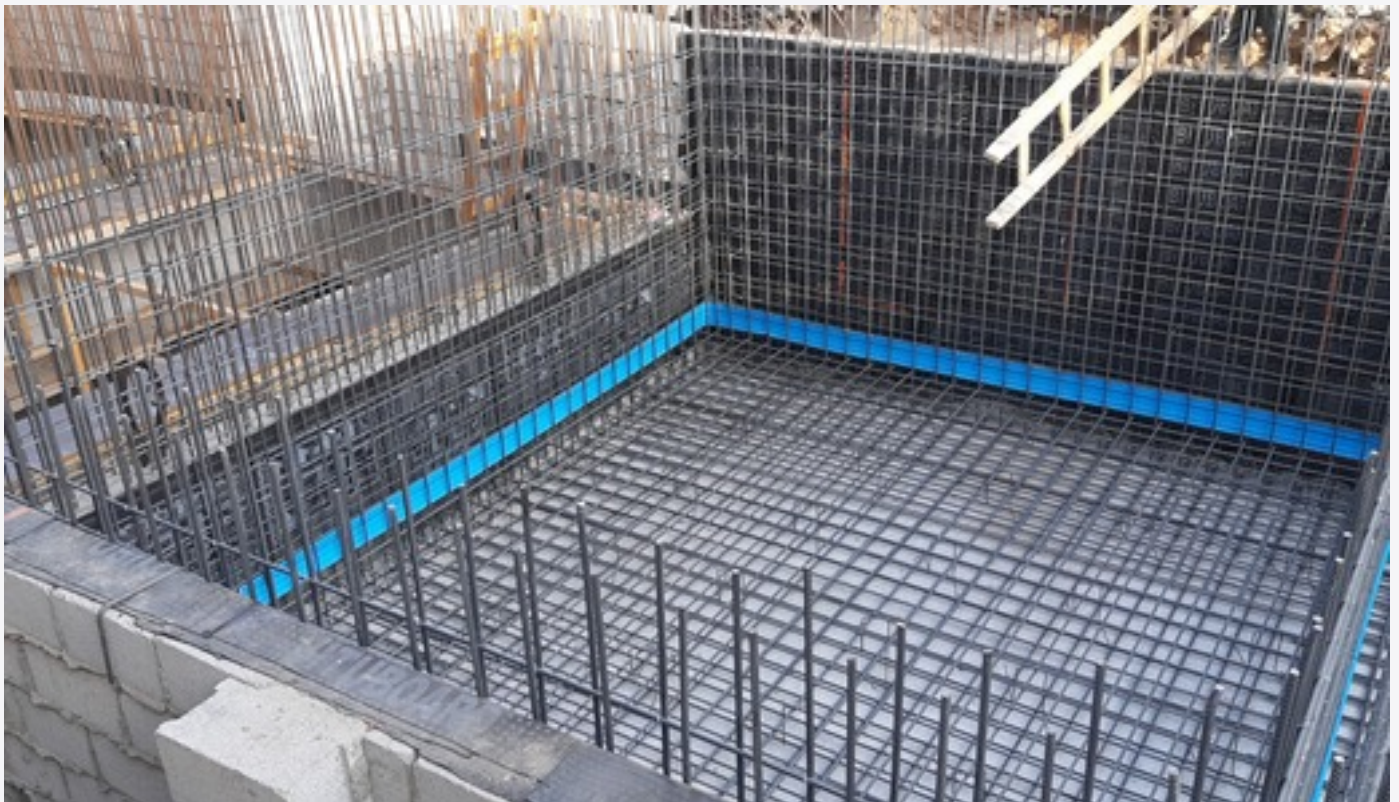
Waterstop Installation - Hamdaniya Tanks
