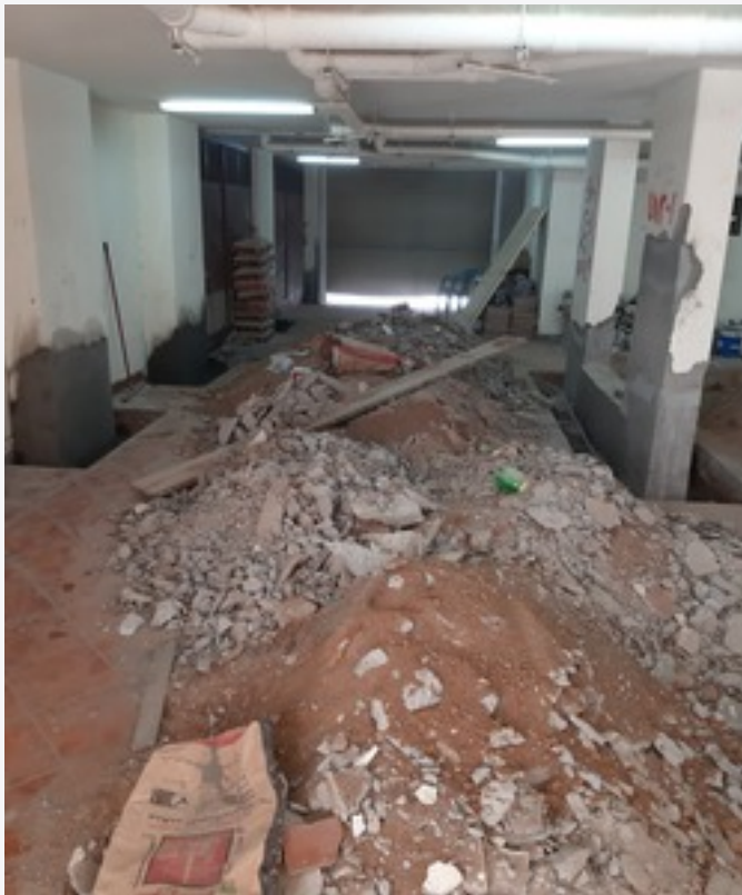
Concrete Repair - Al Salama Buildings
