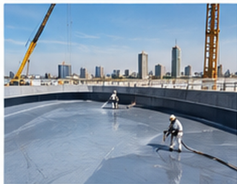
Secondary Containment Lining
