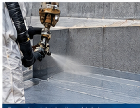
Expansion Joint Sealing with Polyurea
