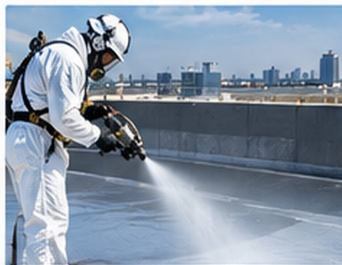
Roof Waterproofing - Polyurea Application
