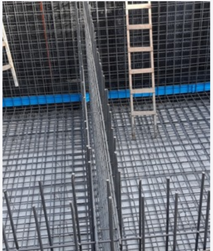
PVC Waterstop - Hamdaniya Tanks
