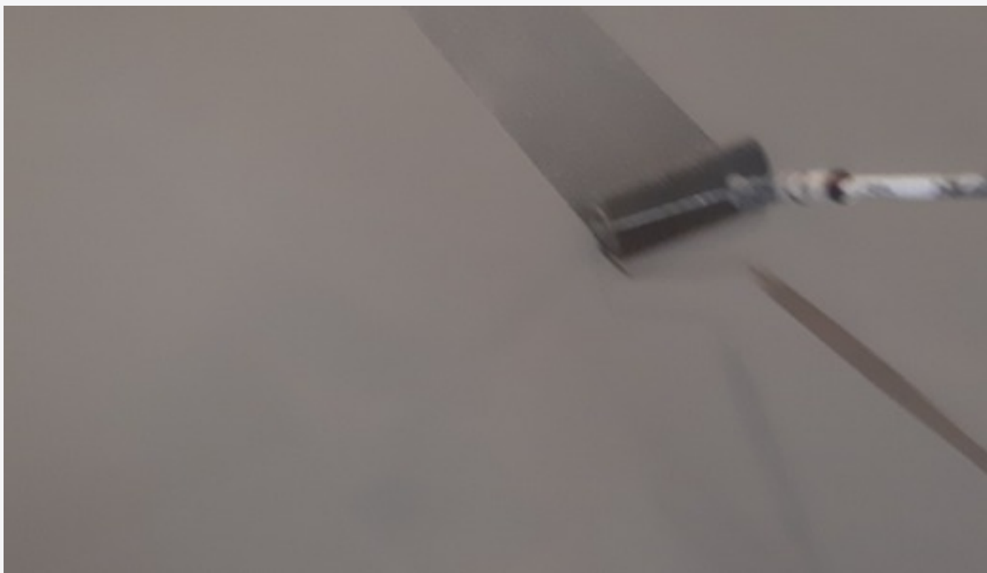
Self-Leveling Epoxy - King Abdulaziz International Airport, Jeddah
